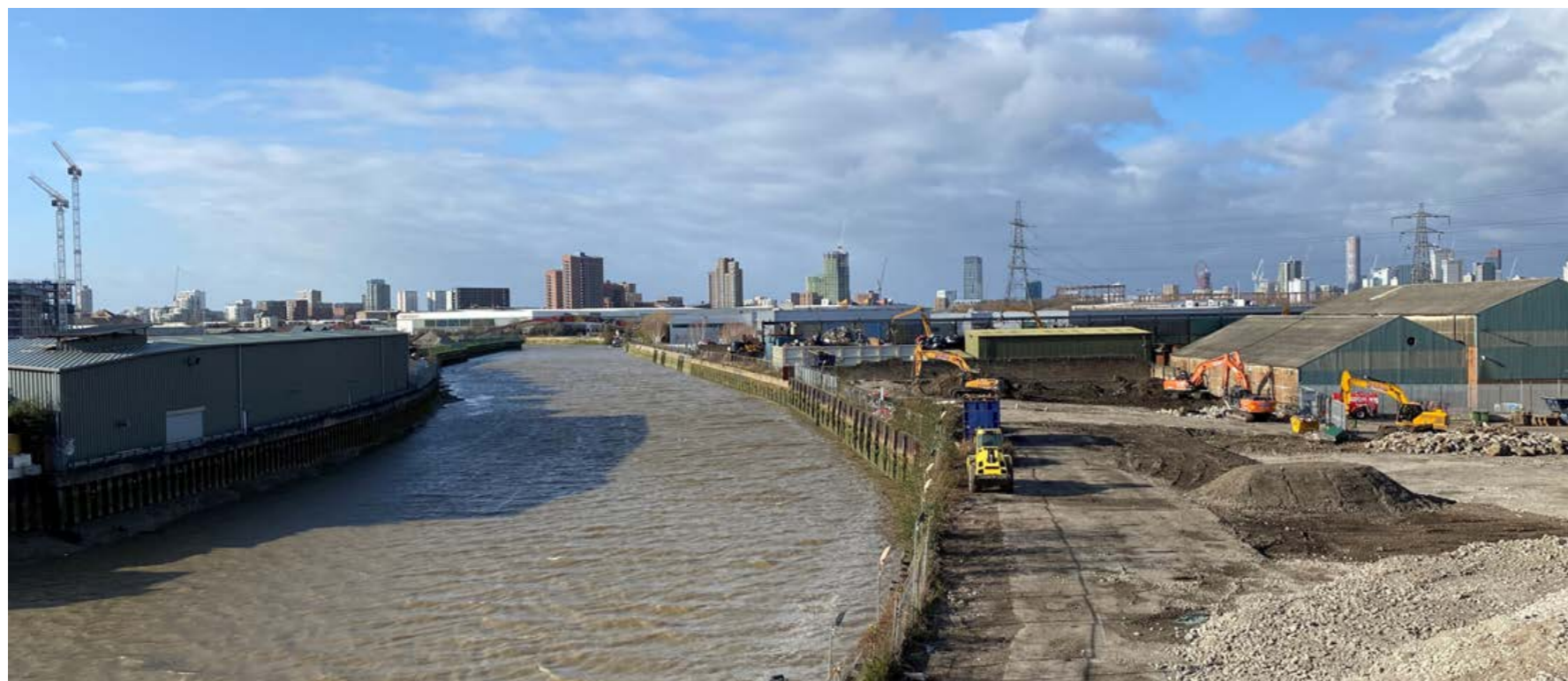
View from A13 looking down the River Lea
